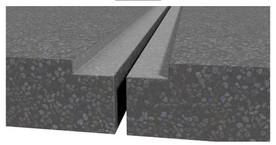
Saw cut topping or concrete deck to prescribed width and depth. Remove concrete from blockout area. Prepare concrete by mechanical means to create a clean sound surface and prime with TuffCrete Primer if required.
