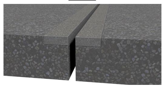
Upon reaching initial set, remove blockout and place PSI backer rod.
