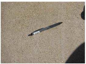
Fig #5 shows concrete with no pinholes or cavities
