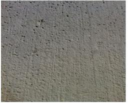
Fig 4 Small Cavities in deck
