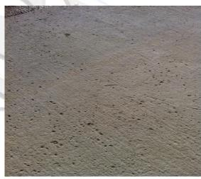
Fig #2 Surface cavities in concrete
